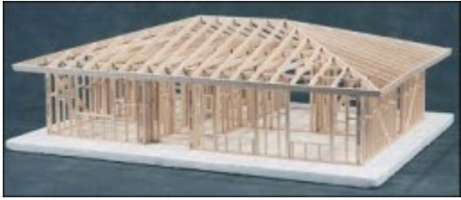
Figure 7-4: Example of a hip roof, which has more slopes than a traditional gable roof
