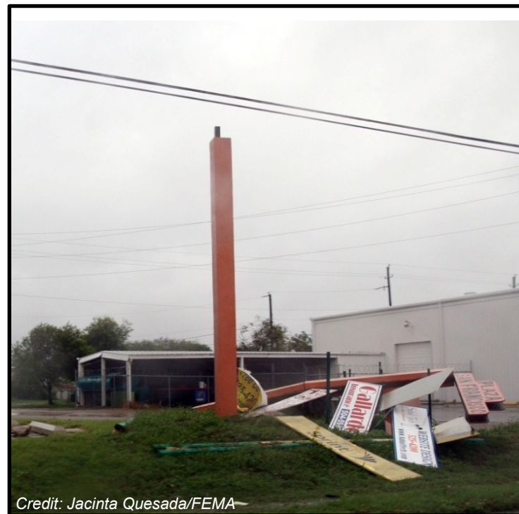
Credit: Jacinta Quesada/FEMA Figure 9-1: A freestanding sign that is damaged by a high wind can potentially cause damage to surrounding areas.
